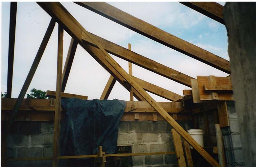
Another pic of the casita roof framing. Anchor bolts hold these wood beams into a concrete beam atop the walls. In this pic, the wood beams are temporarily supported above the formwork as concrete is being poured for the beams. That way everything fits up. The wood to wood connections are thru-bolted.
