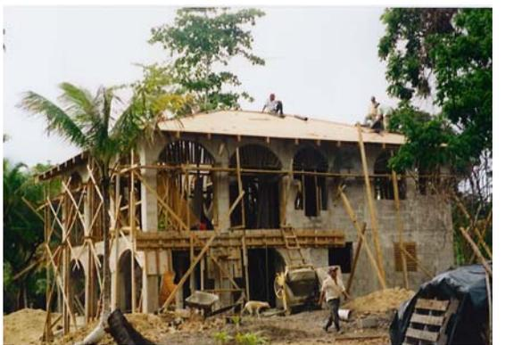
Most of these are views from the beach. The little hill we dug the foundation into is solid limestone as compared to sand which is everywhere else. Most everything is poured concrete except for block fill between concrete columns at the back. Normal construction on the island is wood, so I set-up a concrete apprenticeship program with my workers. This is a very strong house & will survive a hurricane.
