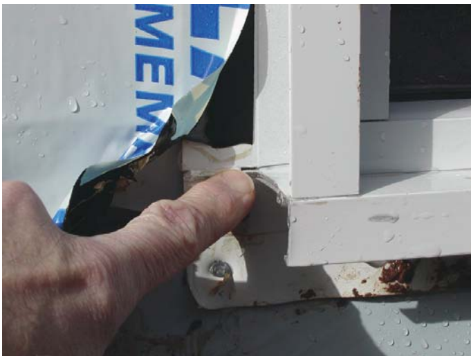
Figure 22: Cracked nailing flange at corner connection
