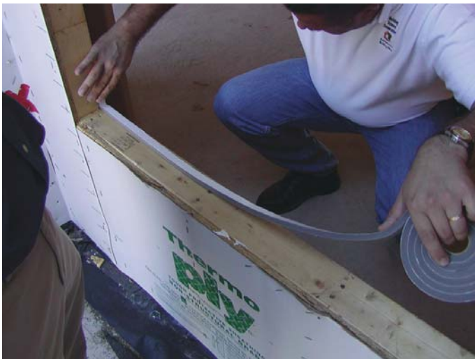
Figure 31: Weather seal gasket used as a backdam
