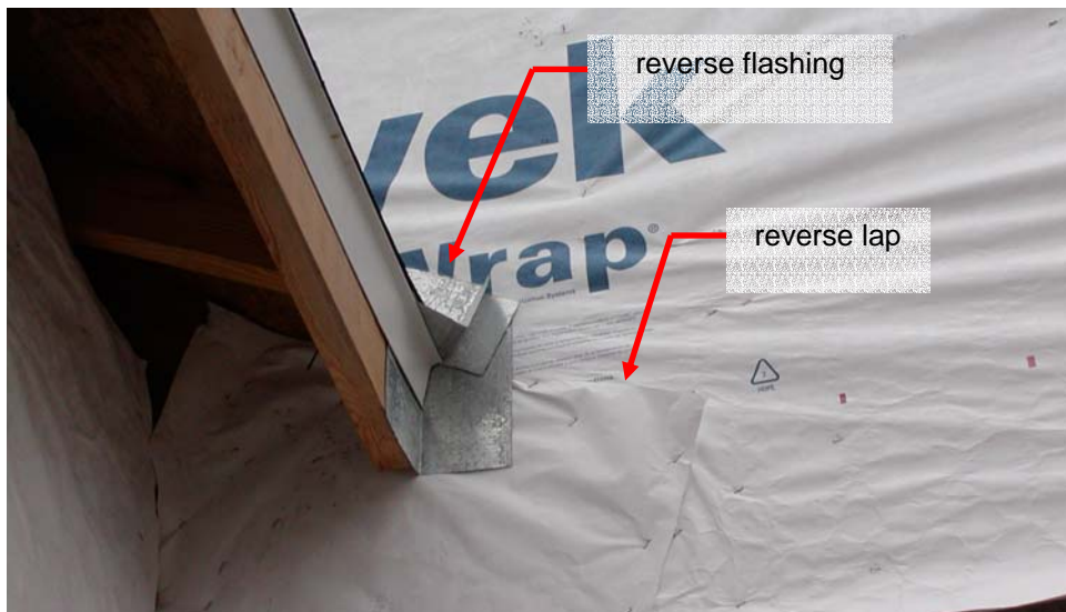
Figure 2: Improper installation of drainage plane materials
