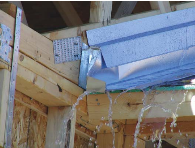
Figure 13: Poorly folded kick out flashing
