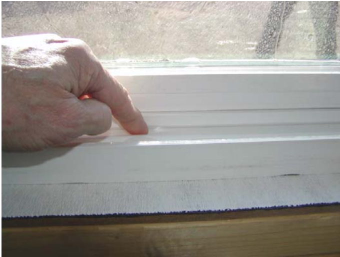
Figure 19: Water intrusion through the window frame
