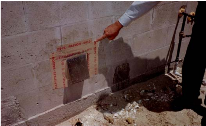
Figure 16: Membrane flashed exhaust vent
