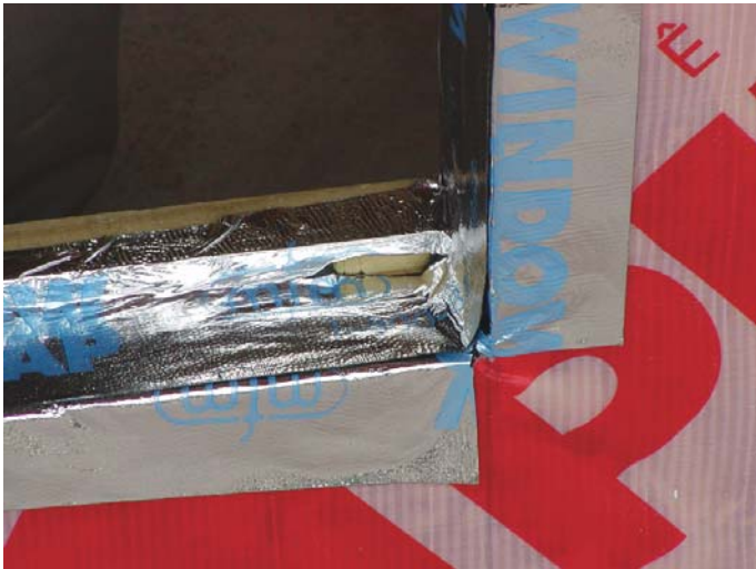
Figure 27: Torn membrane pan flashing
