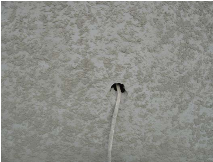
Figure 14: Electrical utility installed after water management system
