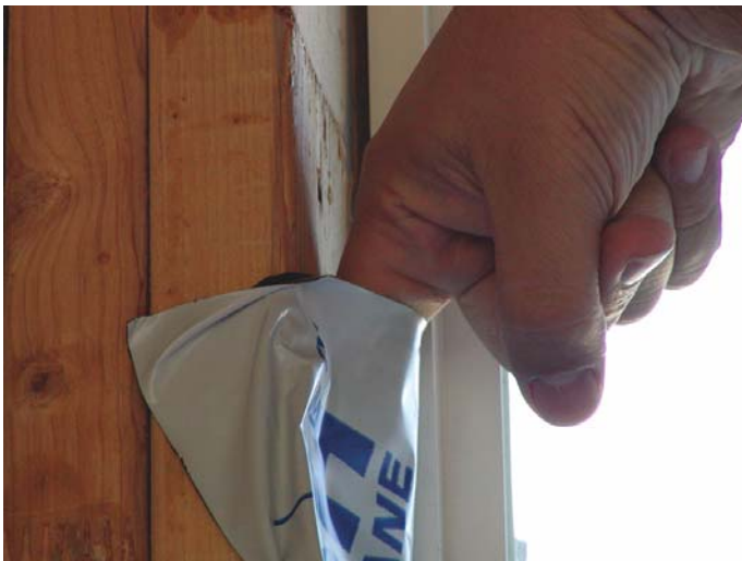
Figure 29: "Fishmouthing" of the membrane
