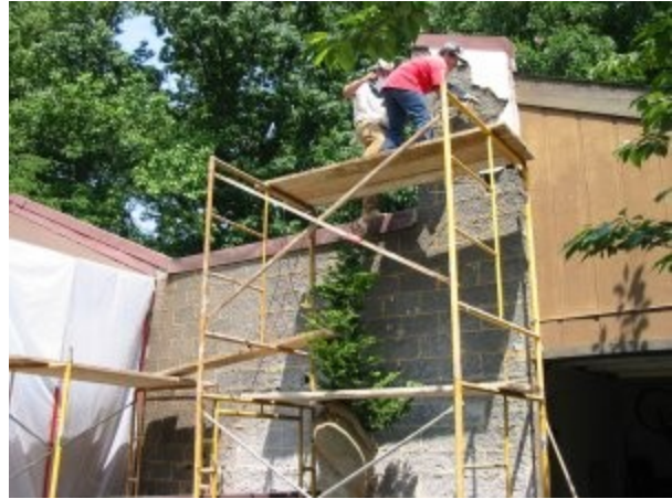
An ounce of prevention is worth 3,000 lbs. of cure. Whole wall is stripped down to block. This assures a nice job. Patches almost always show.
