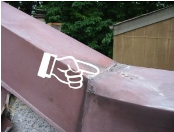
The culprit was this roof cap. Water runs right down the cove in the cap and gets behind the stucco.
