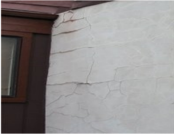
Badly cracked up and loose stucco caused by leaking roof cap
