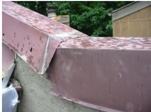
Bottom cap is removed and pushed under the upper cap. The overlap prevents water infiltration. This would have been prevented if the bottom piece was put on first, 30 years ago.
