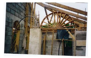
This is how I formed the arches. The black plastic tubing is my electrical conduit inside poured concrete.
