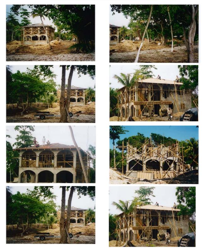
Most of these are views from the beach. The little hill we dug the foundation into is solid limestone as compared to sand which is everywhere else. Most everything is poured concrete except for block fill between concrete columns at the back. Normal construction on the island is wood, so I set-up a concrete apprenticeship program with my workers. This is a very strong house & will survive a hurricane.
